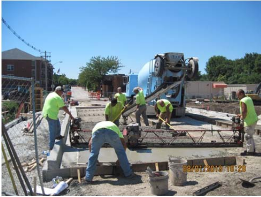
Photo 1: Workers pour north bridge approach pavement.
