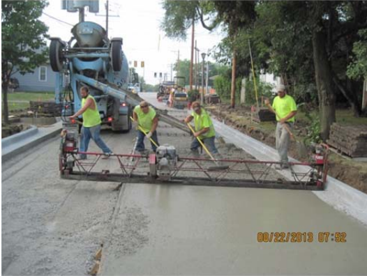
Photo 19: Workers pour pavement on north Race Street.
