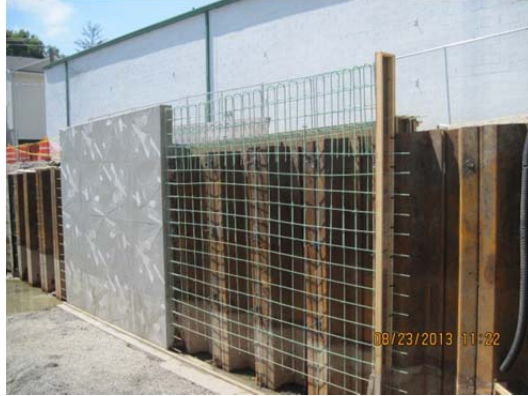
Photo 12: First section of Wall #2 – sedge seed form liner.
