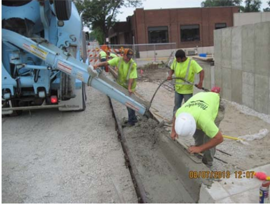
Photo 3: Workers form curb for south bridge approach.
