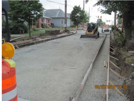
Photo 18: Grading and curb forms, north Race Street.
