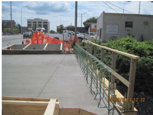
Photo 8: Completed sidewalk for Broadway box culvert repairs.
