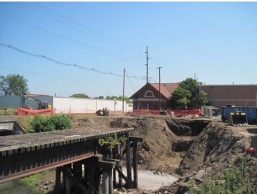
Photo 23: Looking at excavation for east trestle abutment.
