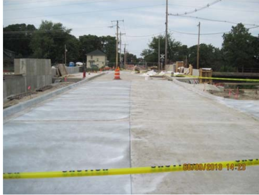
Photo 4: Completed south bridge approach pavement.
