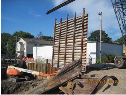
Photo 9: Form placement for first section of Wall #2.
