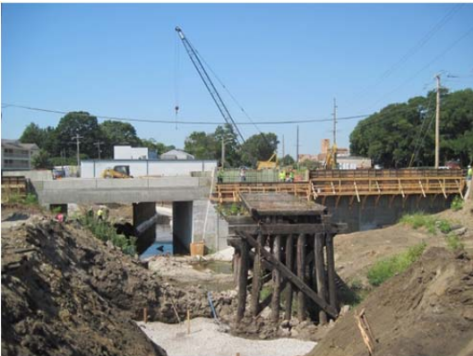
Photo 24: Looking west at trestle and Race Street Bridge.
