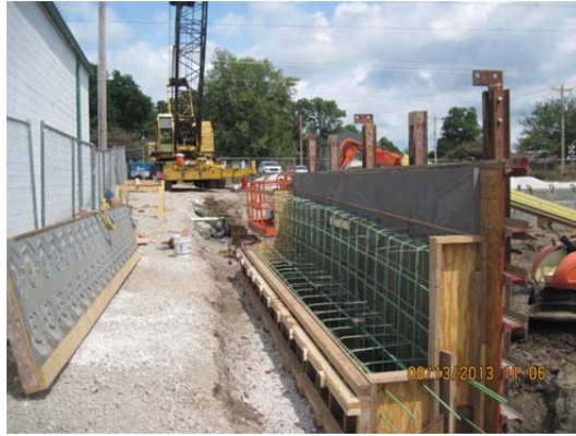
Photo 10: Formwork and rebar for first section of Wall #2.
