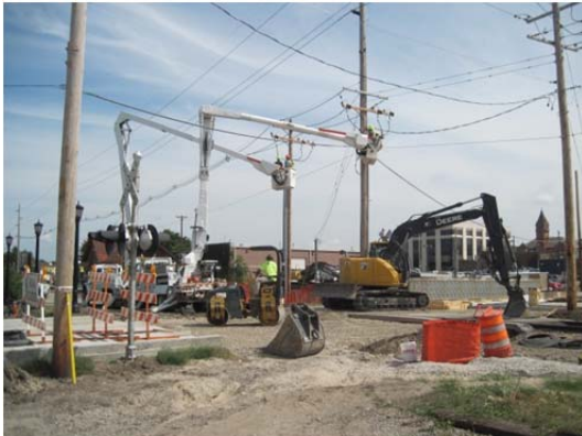
Photo 13: Ameren power relocations through bridge.
