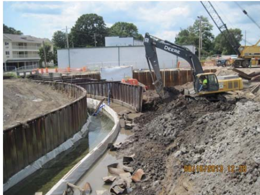
Photo 14: Channel sheeting removal on north side of creek.
