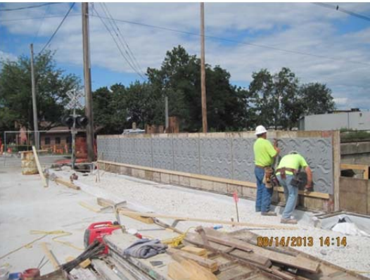
Photo 21: Workers form parapet wall off NE corner of Race Street Bridge.
