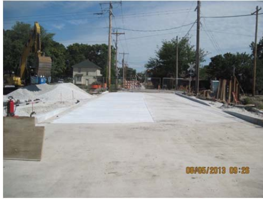
Photo 2: Completed north bridge approach pavement.
