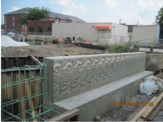
Photo 11: Completed parapet for first section of Wall #2.
