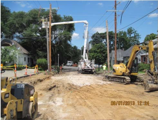
Photo 17: Utility relocation and demo on north Race Street.
