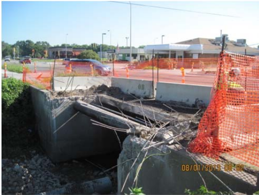
Photo 5: Demolition for Broadway box culvert repairs.
