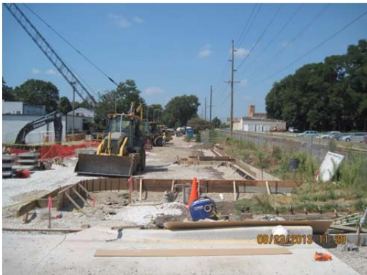
Photo 15: Curb & gutter forming for City Parking Lot #25.
