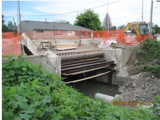
Photo 6: Falsework for Broadway box culvert repairs.
