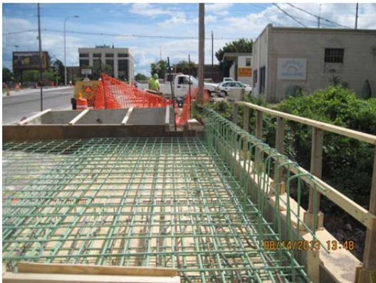
Photo 7: Rebar for west Broadway box culvert repairs.
